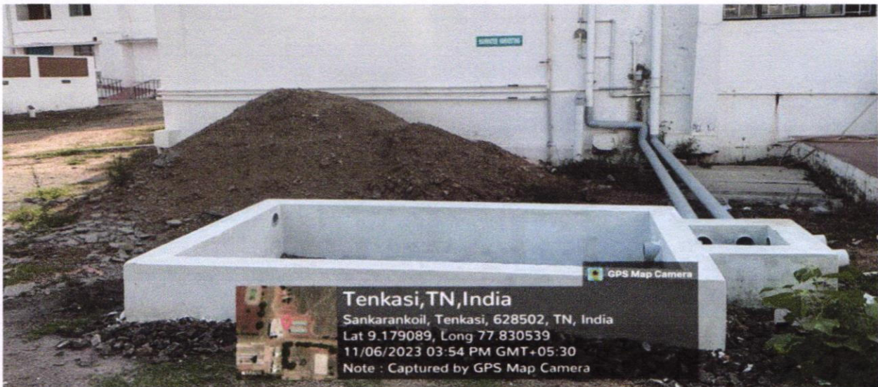
Rain water harvesting tank 2 at college backside
